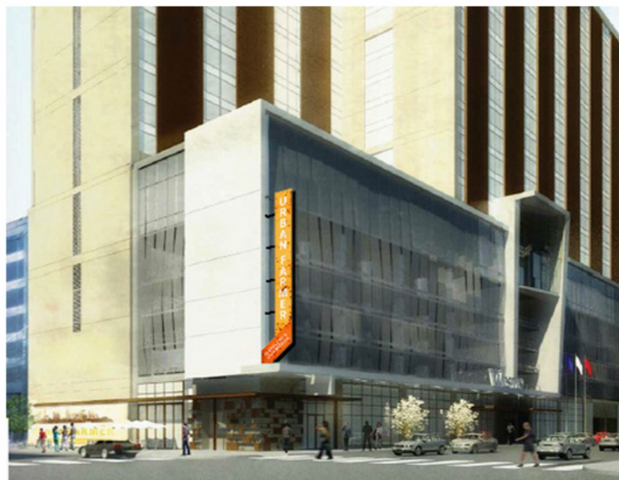
A rendering of what Urban Farmer, Cleveland's Steakhouse and the new Westin will look like.
